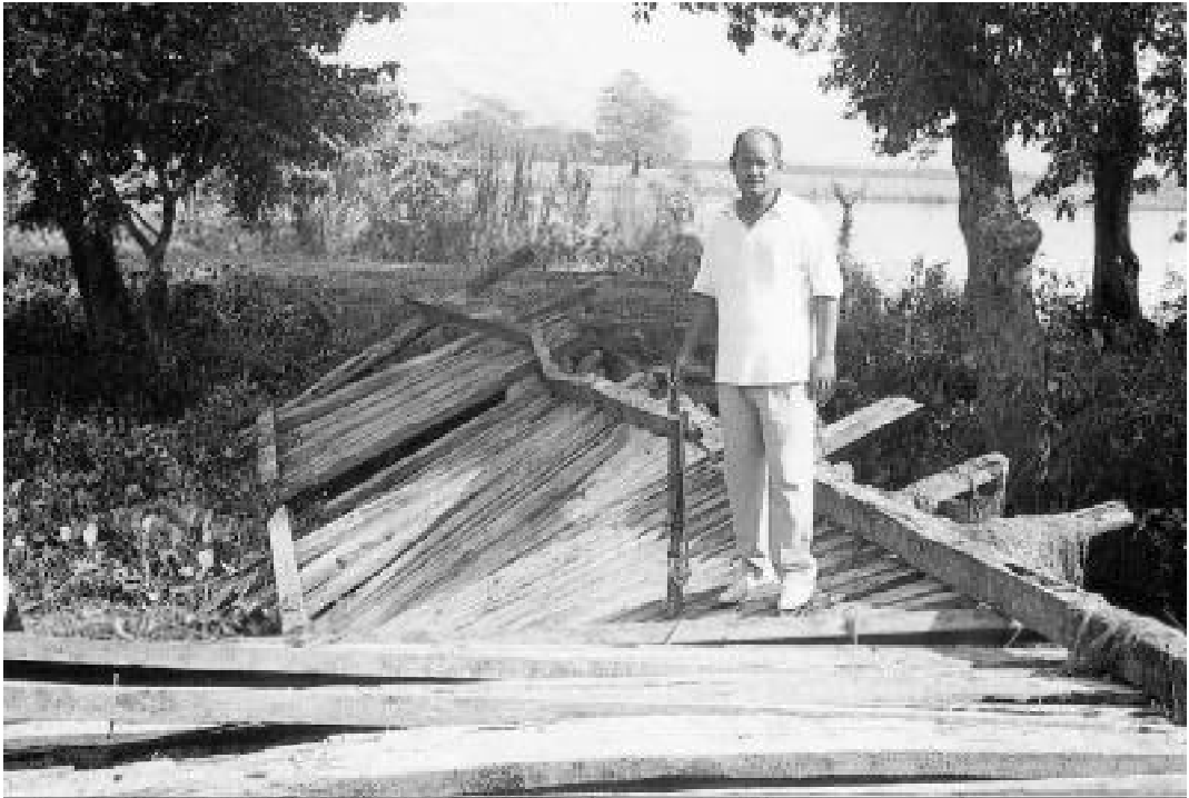
A damaged bridge with Mr D. Boro, the Range Officer in central Kaziranga.
